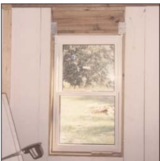
17. WINDOW DETAIL: (Pic. 011)
