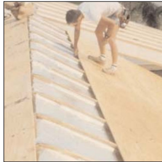
10. COMPLETING ROOF DECKING: (Pic. 008)
