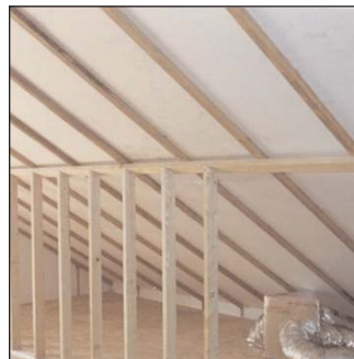
15. INSULATED ATTIC: (Pic. 024)
