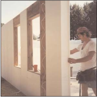
5. WALL ASSEMBLY ON SLAB (Pic. 016)
