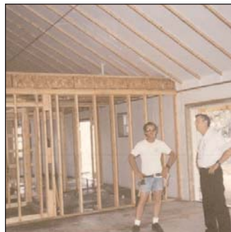
14. DRY-IN INSPECTION: (Pic. 031)
