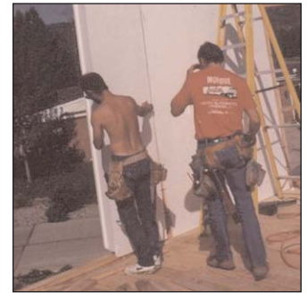
4. WALL GOING UP: (Pic. 005)
