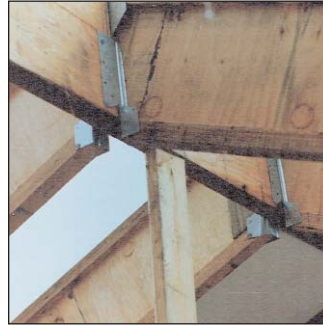
7. RAFTER/RIDGE DETAIL: (Pic. 030)
