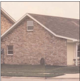
13. BRICK AND SIDING: (Pic. 021)
