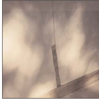
6. SLAB TO STUD ANCHORS: (Pic. 006)
