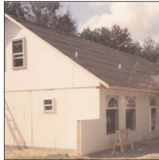
11. COMPLETED SHELL: (Pic. 050)
