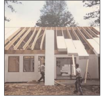
8. INSERTING ROOF BEAMS IN TJ'S: (Pic. 013)
