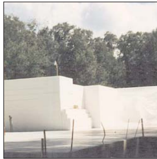
2. PANELS READY ON SLAB W/ANCHORS: (Pic. 009)
