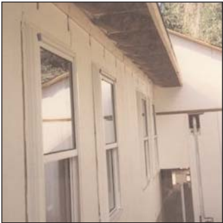
9. RAFTER-TO-STUD STRAPS: (Pic. 048)
