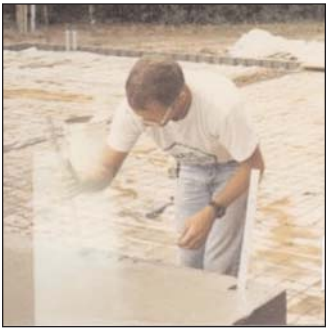
1. PLACING ANCHORS IN WET SLAB: (Pic. 010)
