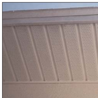
18. VENTED SOFFIT: (Pic. 029)
