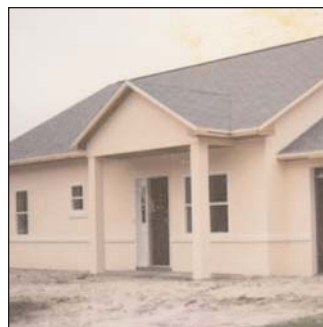
19. STUCCO FINISH: (Pic. 027)
